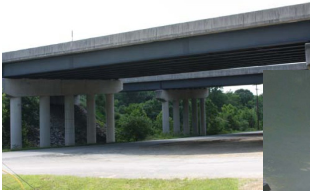
3-span steel girder bridge (08/18/09 - Roanoke)
